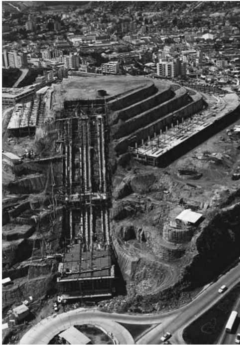
The hill known as La Roca Tarpeya was sculpted to fit El Helicoide. On its northern flank, four state-of-the-art elevators were to be installed. Photo Estudio Jacky. Courtesy Bornhorst Archive.
